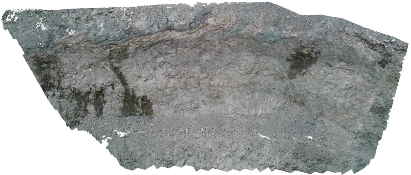
Fig. 3 Orthophoto of the north-eastern pit wall looking north.
