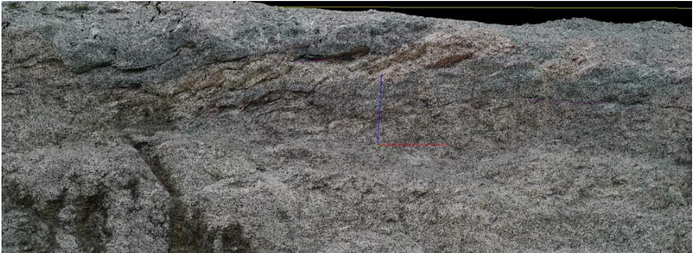
Fig. 5. Coloured 3D point cloud generated by aerial photogrammetry for wall mapping.
