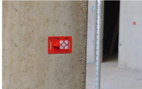
Figure 5 - Survey tags can be used as fixed and accurately localized benchmarks.
