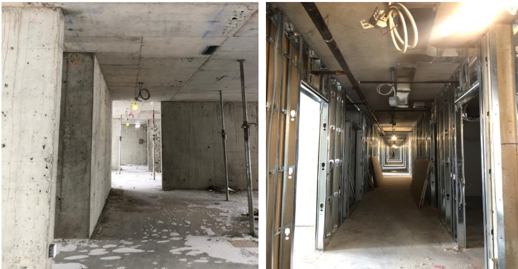
Figure 3 - Formed and stripped floor hallways before and after drywall erection.
